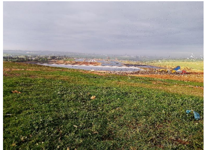
Figure 1. Leachate storage basins at the Oum Azza landfill
