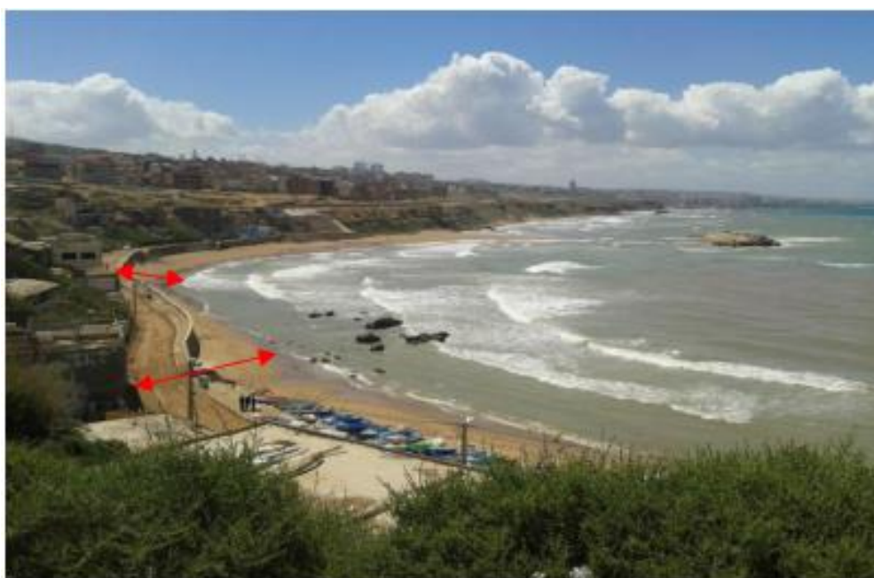
Figure 12. Coastal linear urbanization in Sidi El Majdoub threatening the 300 m zone (Photo by Kies, 2018)
